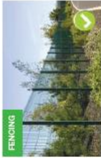
GLD Fencing Exempla 1.2m high weld mesh panel fencing - green or similar approved
